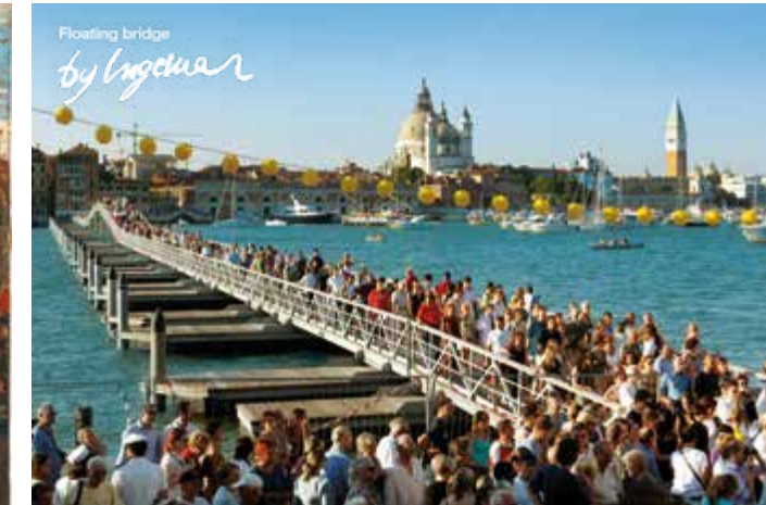
The temporary floating bridge on pontoons built by Ingemar, since 2002
