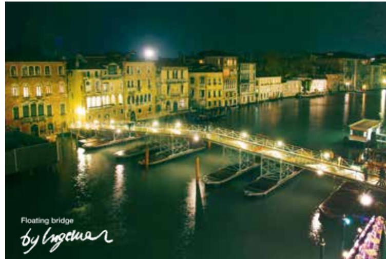
The floating temporary bridge on pontoons built by Ingemar on the Grand Canal
